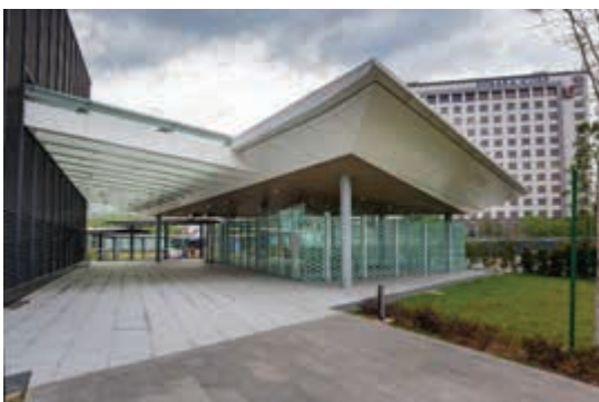
Tun Razak Exchange Station
