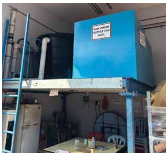
New Rainwater Harvest Collection System
